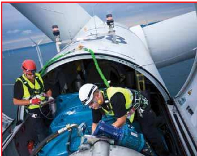
Routine maintenance performed up-tower (courtesy of Siemens)
