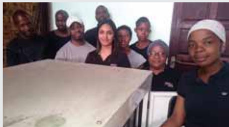
The WearCheck Middelburg team is proud of their brand new generator, which protects the laboratory equipment from interrupted power supply such as load shedding. They are, from left to right, Caven Selane, Siphon Magcaba, Rufus Mathekgane, Robinson Tshabalala, Salisha Dhanasar, Nelly Dlamini, Pateince Skosana, Julia Motshwene and Randy Mathibela
